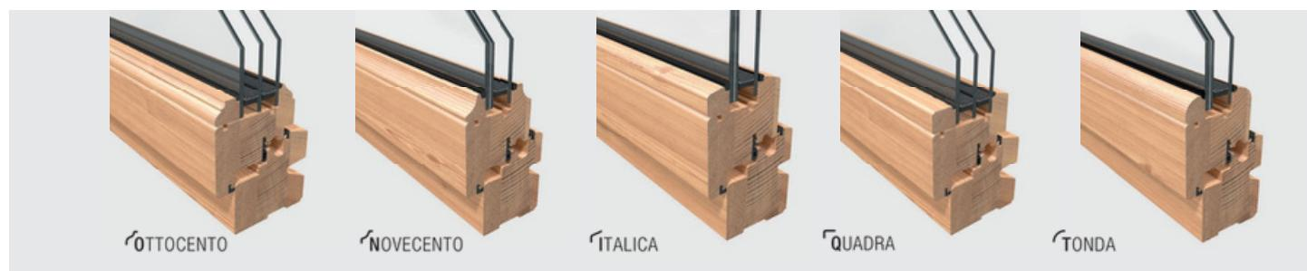
**OUTSIDE** The external wood style is determined by the shape of the glazing bead and is available in the following versions:
